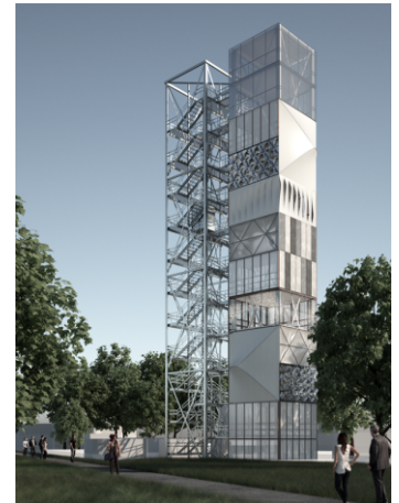
The adaptive structural elements are currently being tested in practice in a demonstration building. The adaptive high-rise building, which is approximately 37 metres high, is located on the campus of the University of Stuttgart. (Photo: ILEK, University of Stuttgart)
